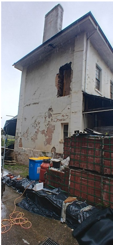
rear wing - south-west corner
